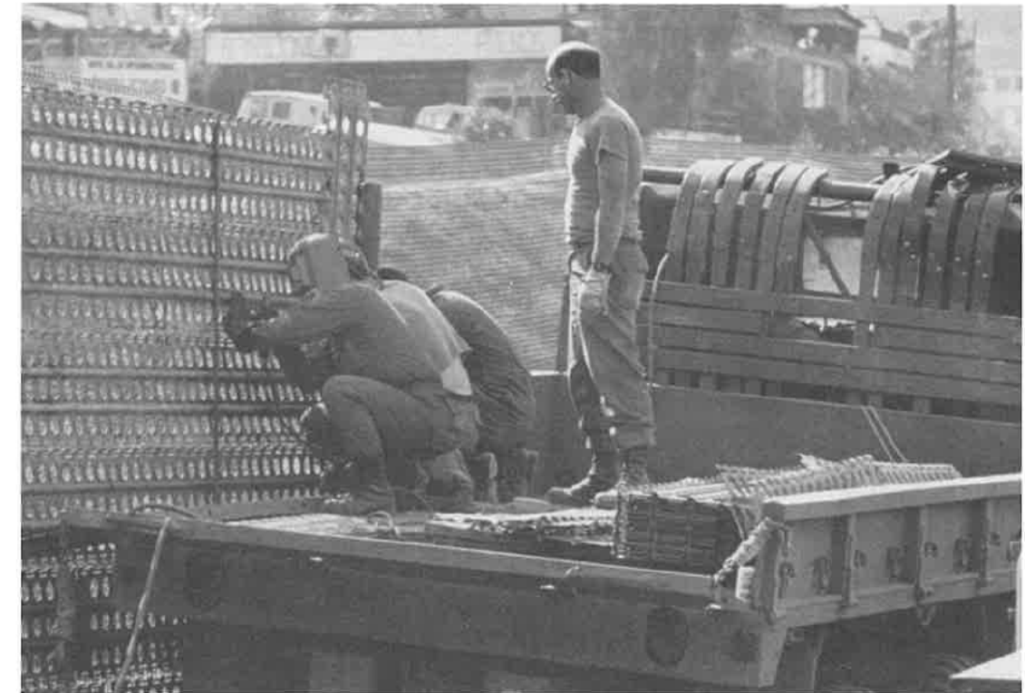
Military Reservists reinforce border fence near San Diego with surplus metal used for temporary landing strips. The fence repair was a cooperative project of the Border Patrol and the Department of Defense in support of overall border enhancement.
